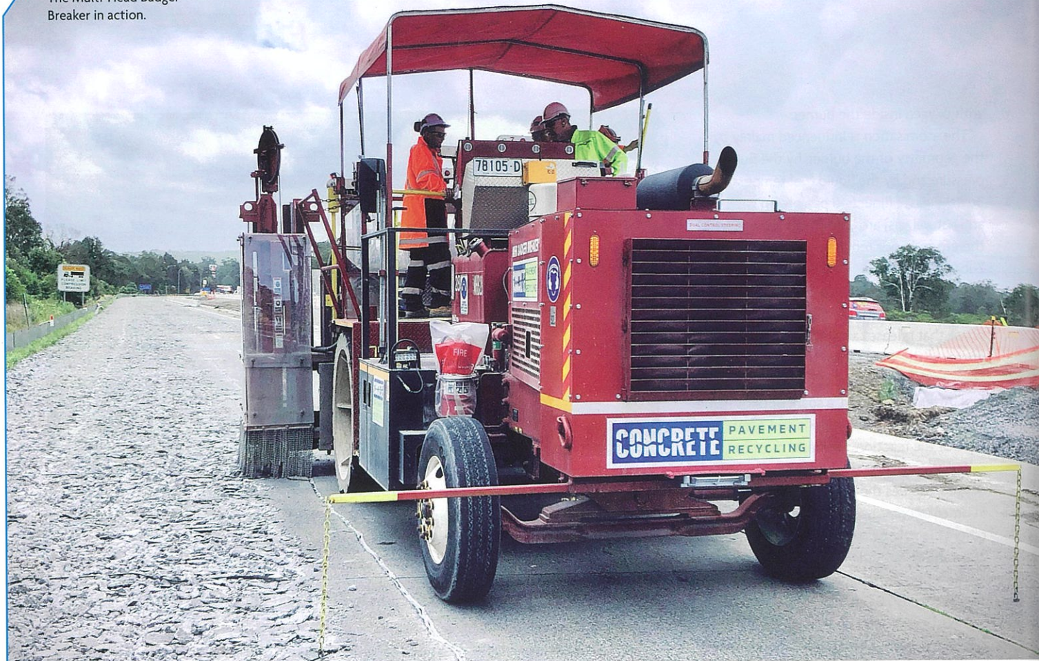
The Multi-Head Badger Breaker in action.
